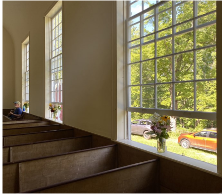
Beautifully restored windows that function!
